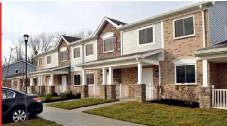
BUILDING #15 AT WINDCLIFF VILLAGE PHASE II
