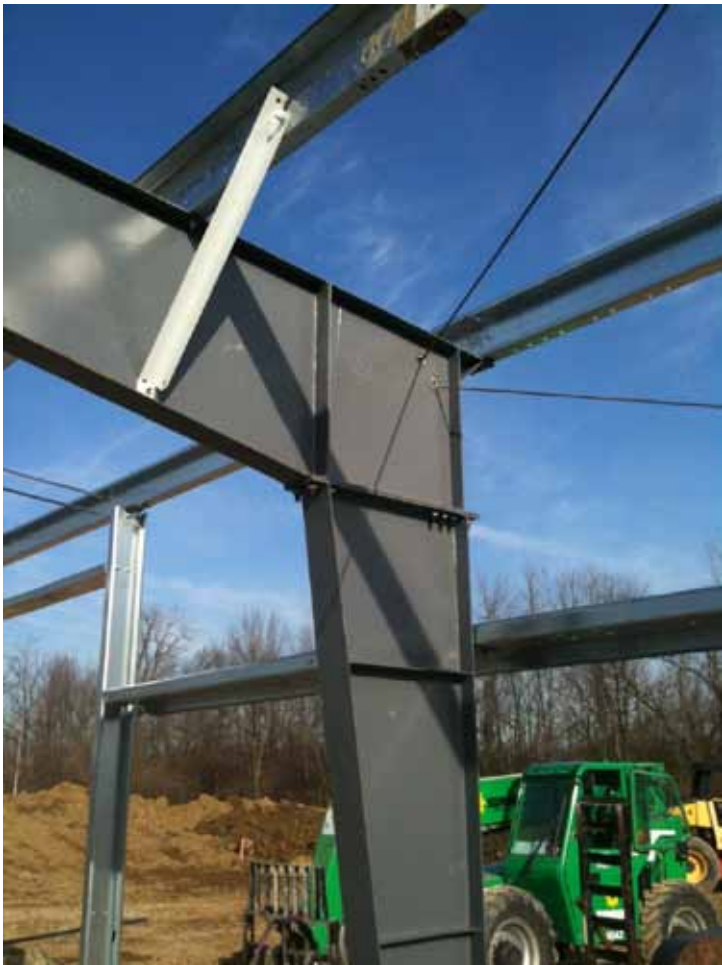
Butler® Building Pre-Engineered Structure Being Erected —Courtesy of Bill Hibner
